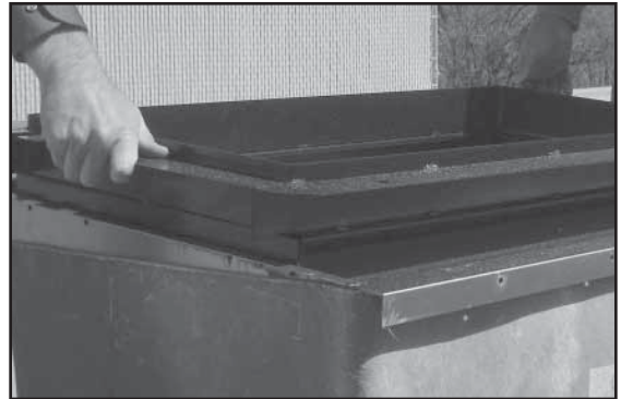
Figure 17 - Installing Metal Top
