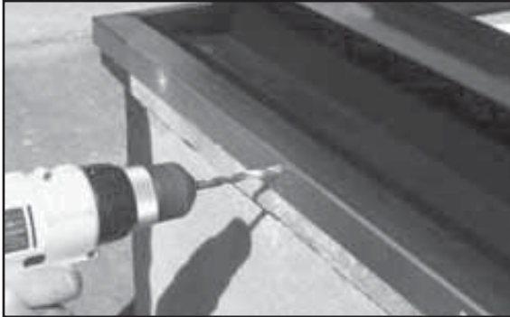
Figure 1 - Drilling into Metal Frame
