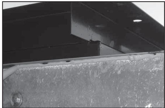
Figure 28 - Applying Sealant to Sump Top
