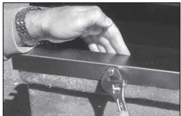
Figure 6 - Tightening Bolts
