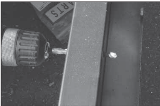
Figure 19 - Drilling Through Metal Frame
