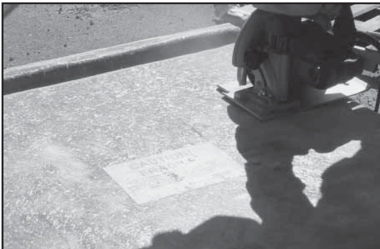
Figure 15 - Cutting Down Sump
