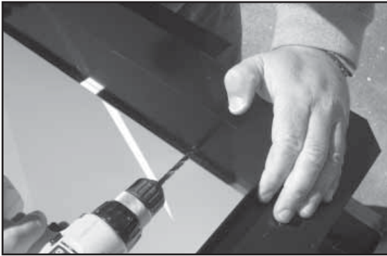
Figure 7 - Drilling from the Inside of the Sump
