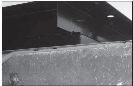
Figure 11 - Applying Sealant to Sump Top
